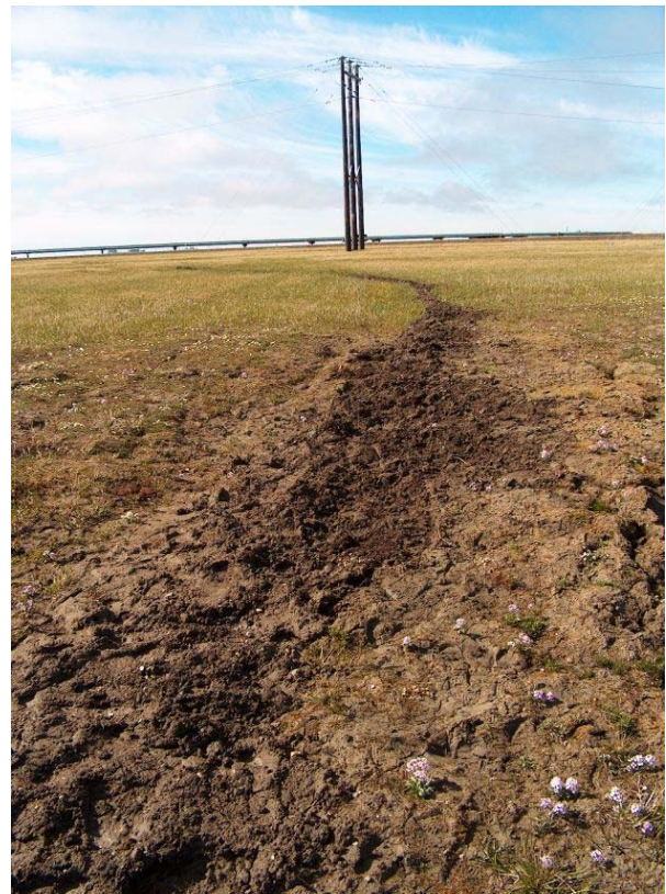
Trench remediation, NE Pad L3, North Slope.
