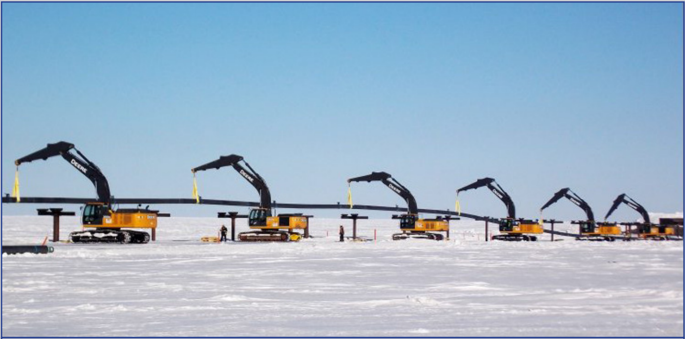
Construction of Point Thomson Export Pipeline completed in 2014. In the image above crews lift the pipe on to the installed vertical and horizontal support members. Photo courtesy of ExxonMobil
