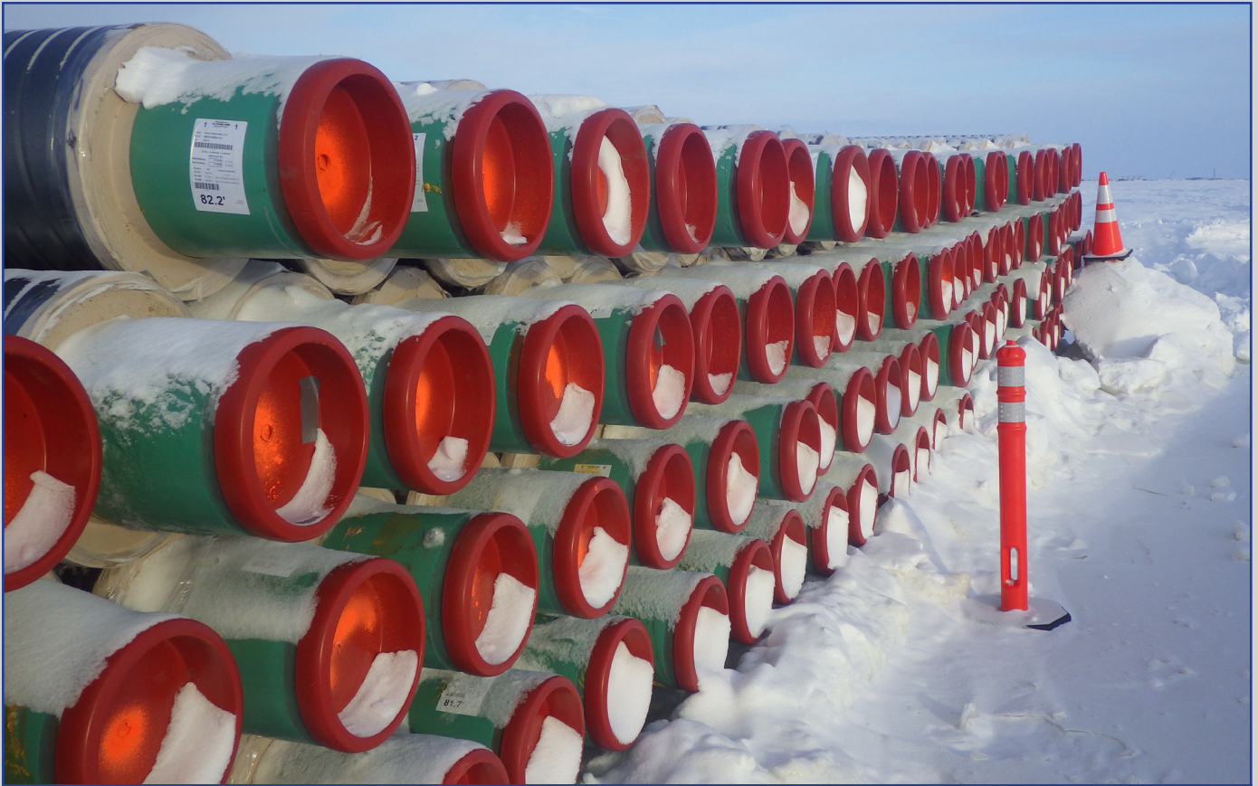
Piping staged for the construction of Point Thomson Export Pipeline
