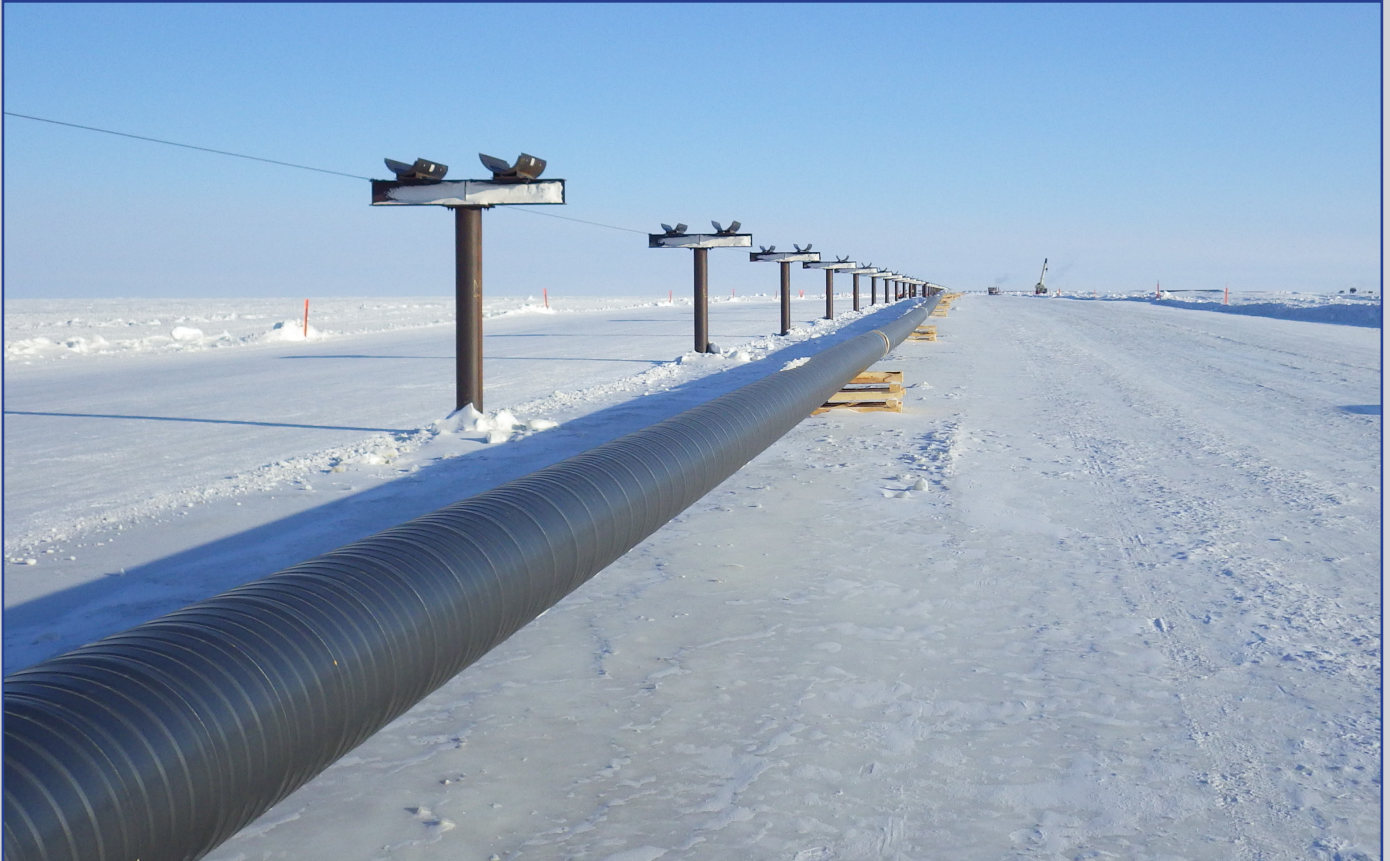
Point Thomson Export Pipeline prior to being raised on to the VSM pipe saddles
