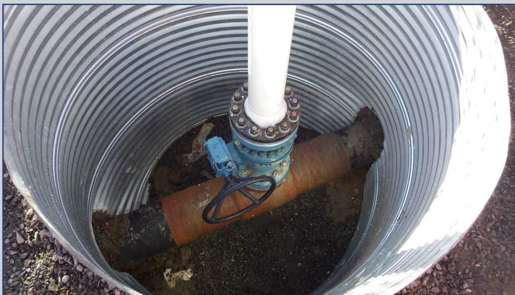
Bart Pad lateral tie-in to Kenai-Kachemak Pipeline
