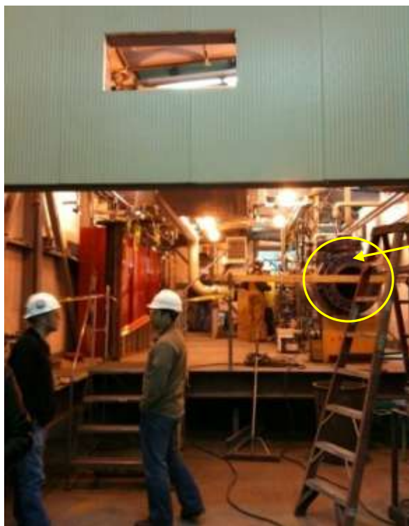
Figure 54: CPF-1 Pig Receiver Module
