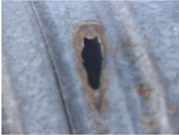
Figure 46: Perforation of Insulation
