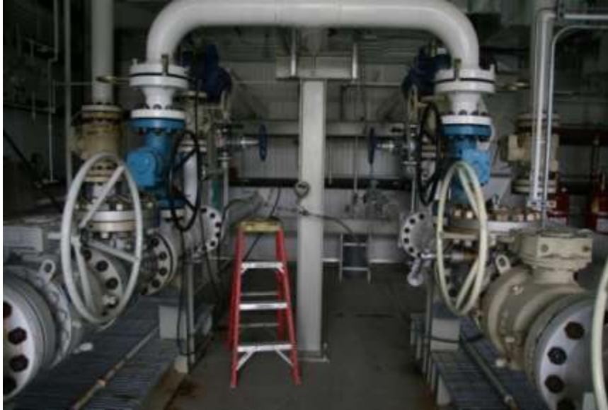
Figure 34: Inside the KKPL Terminus; Two Tested Spring Valves
