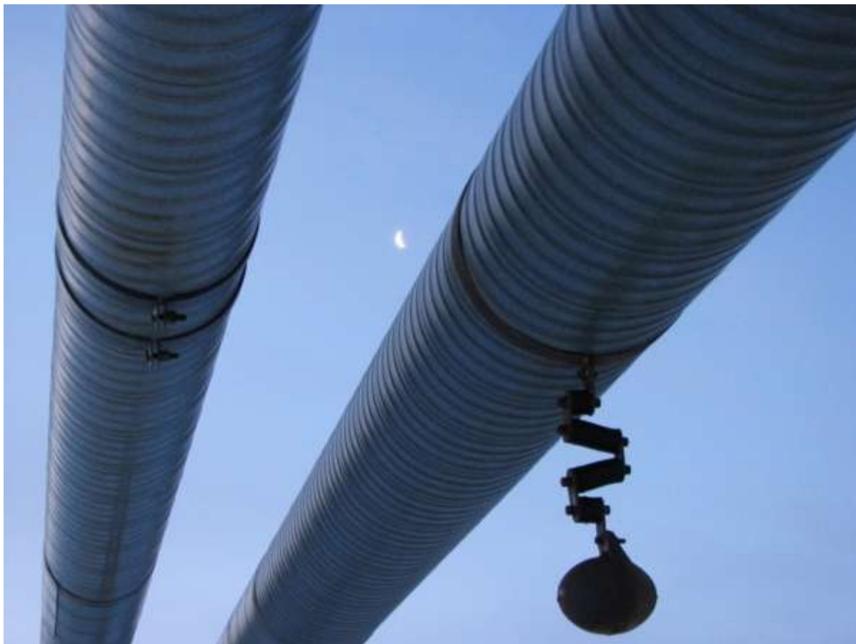
Figure 45: Vibration Dampener on the Milne Point (oil) Pipeline
