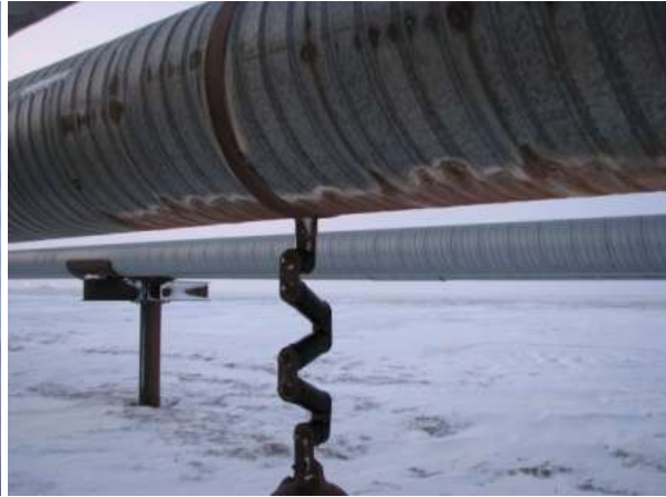
Figure 47: Significant Rust
