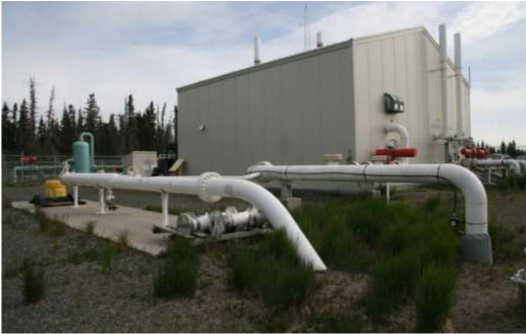
Figure 31: Pig Receiver and KKPL Terminus Building
