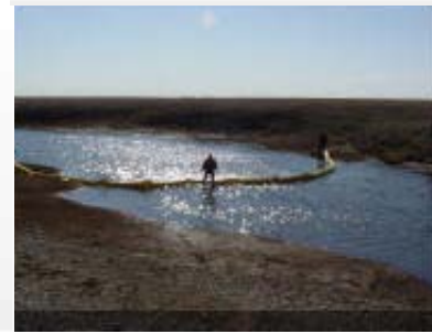
Spill Drill – Booming a River
