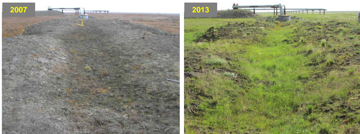
Figure 2. Views (facing east) of backfilled trench, Badami Pipeline East Shaviovik Crossing, 13 September 2007 and 3 August 2013.
