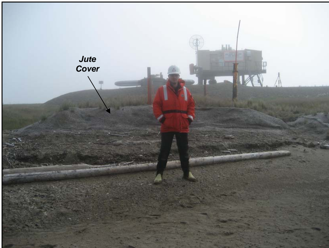
Photo 1. Jute Fabric Cover and Driftwood Debris at Shore Crossing
