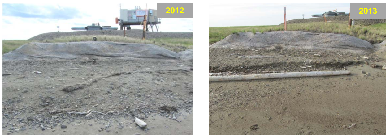
Figure 4. Views (east) of side slope treated with erosion control matting, Northstar Pipeline Landfall Shore Crossing, 28 July 2012 and 3 August 2013.
