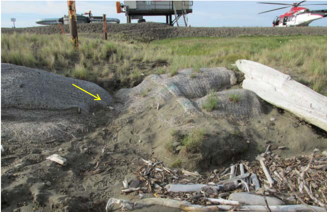
Figure 5. Close-up of area at west end of erosion control fabric where a slight gully has formed (yellow arrow), Northstar Pipeline Landfall Shore Crossing, 3 August 2013.
