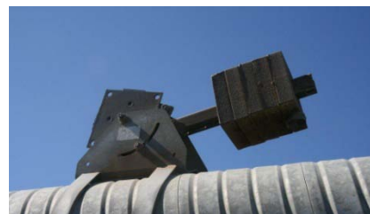
Tuned Vibration Absorber
