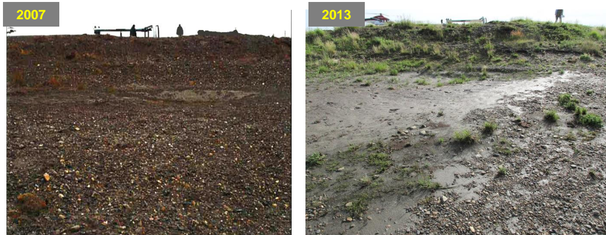
Figure 4. Views (facing east) of the face of the backfilled trench where it meets the river bank, Badami Pipeline East Shaviovik Crossing, 13 September 2007 and 3 August 2013.
